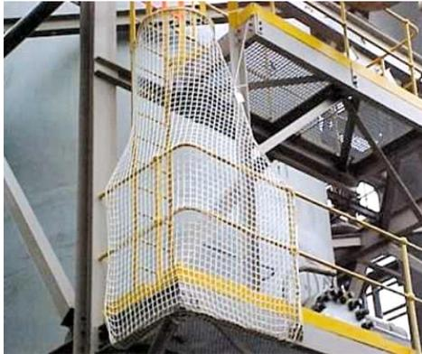
The 'Ladder Netting Safety System' is a patented yet simple and cost effective solution to the problem of vacant space between the first rung of a back scratcher and the deck. This solution can also be applied on ladders where the gap between back scratcher rungs is excessive.
